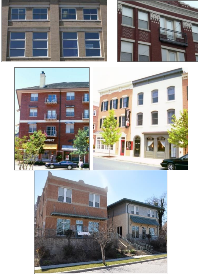
Images showing appropriate window and door designs and proportions for commercial and mixed use buildings.
