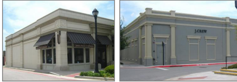
Images showing the side and rear façades buildings finished to match the color and materials of the front facades
