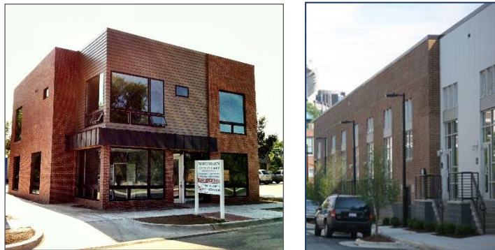
Images of appropriate building materials in the Downtown Edge, Transit Village Edge, Cotton Mill Core, and Cotton Mill Edge Character Districts
