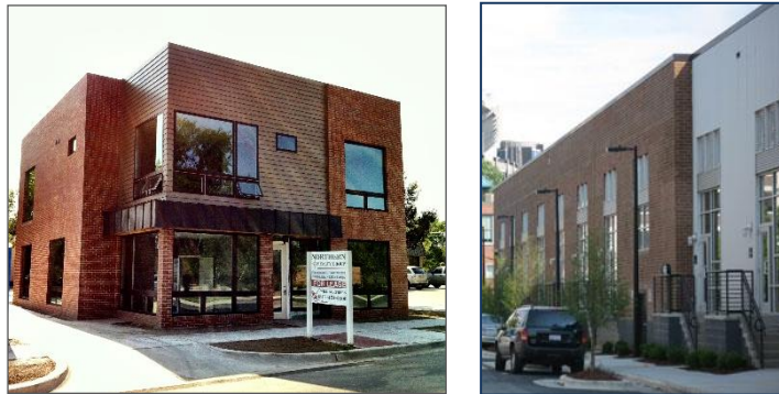
Images of appropriate building materials in the Downtown Edge, Transit Village Edge, Cotton Mill Core, and Cotton Mill Edge Character Districts
