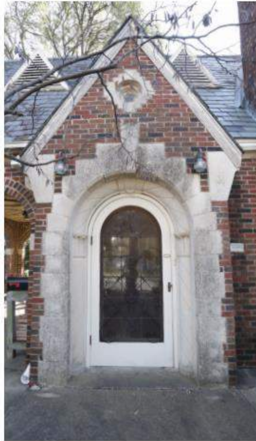
Cut stonework around door opening
