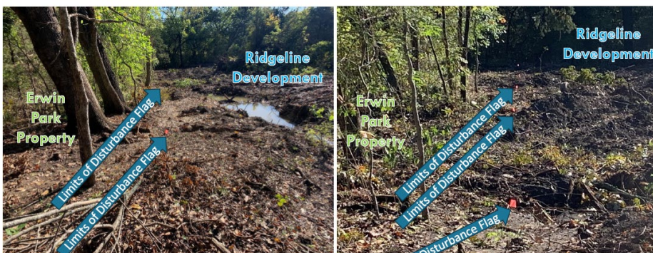
Survey flags showing limits of work (2-5' inside the property line)
