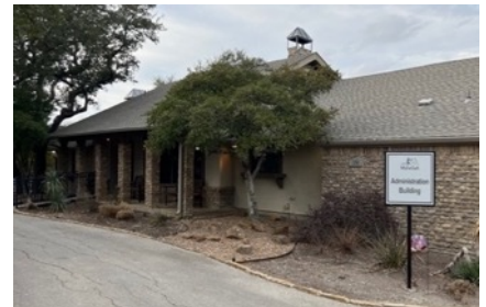
Old 2,200 square foot Admin Building
