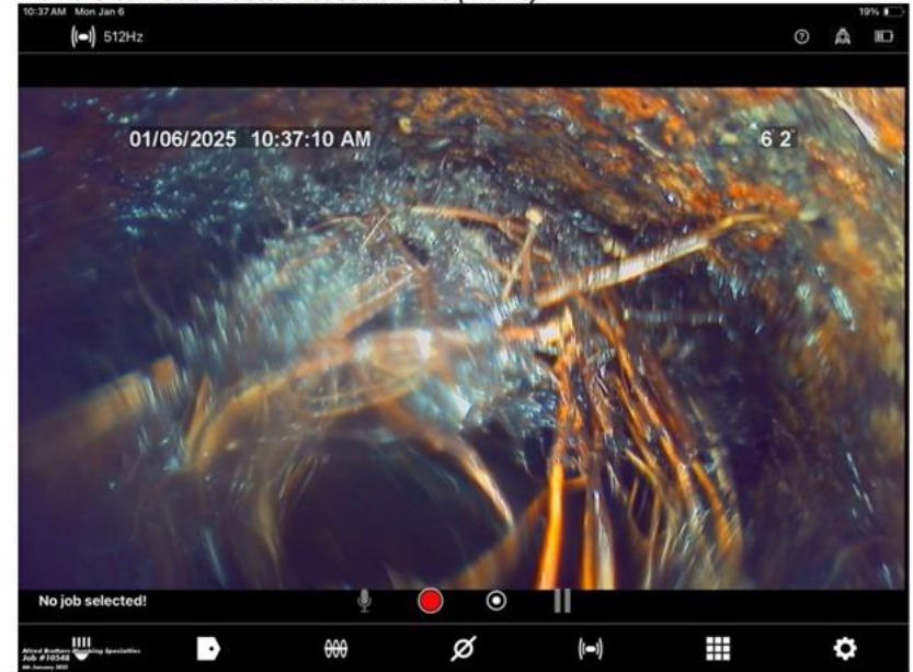
1-6-25 Clean Out: Roots in cast iron line (1-6-25)
