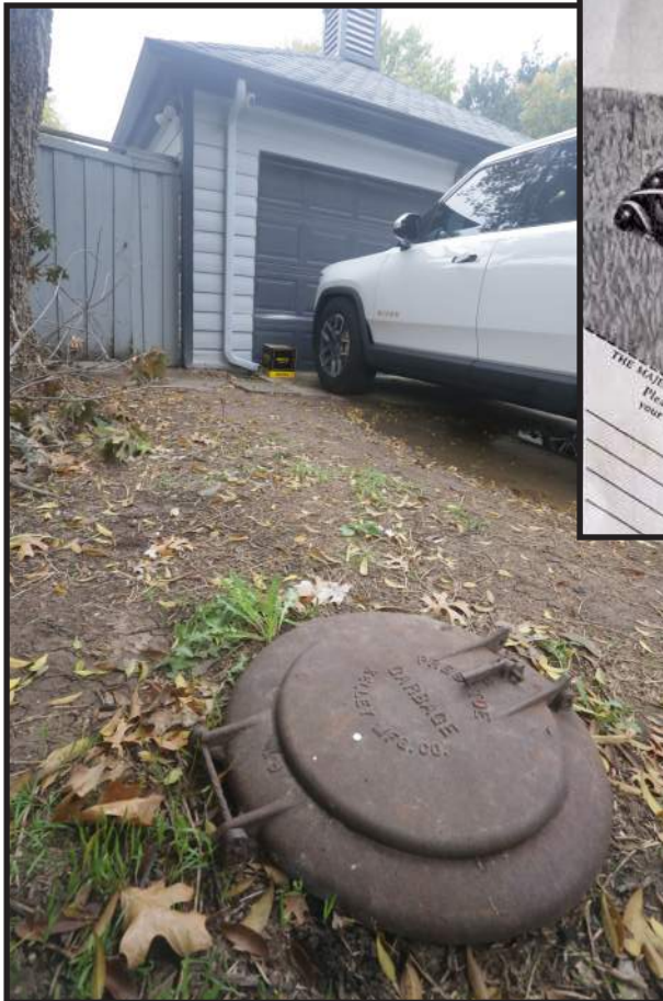
Sunken trash can
