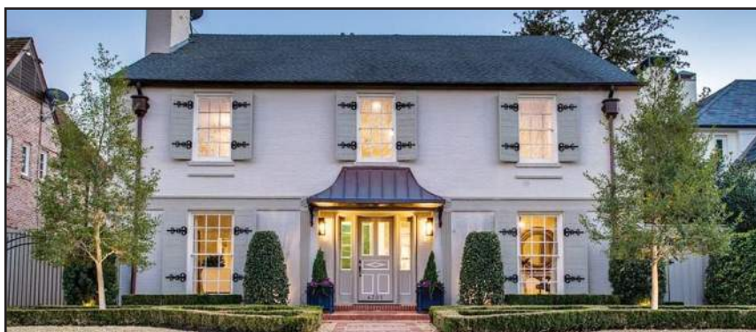
4305 Westway Ave., Dallas TX - 1937
