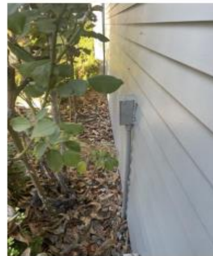
705 N College St #5 (Garage Drainage).
