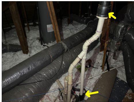
Attic: Cast iron vent conversion to pvc
