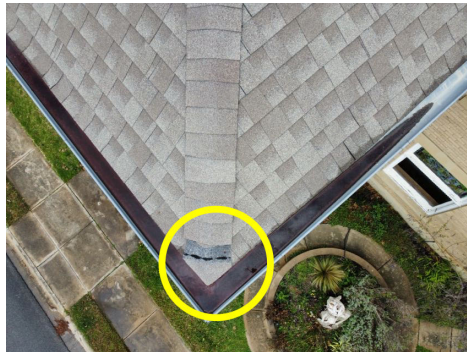
Shingle damage
