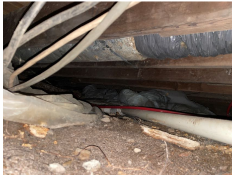
General Crawlspace picture
