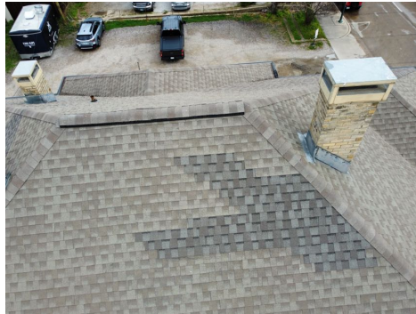
Previous repairs to roofing materials
