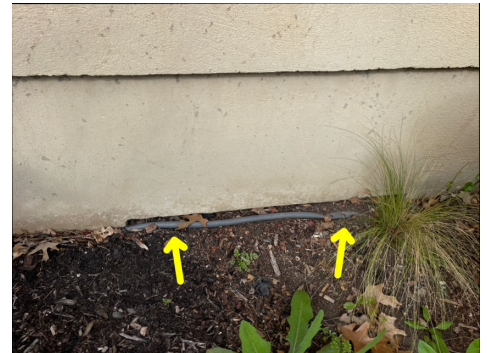
East Exterior: Possible crawlspace vent covered
