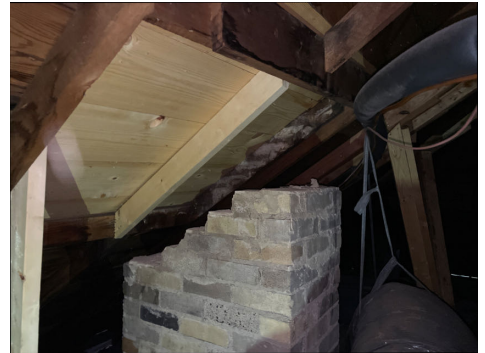
Attic: Chimney terminated
