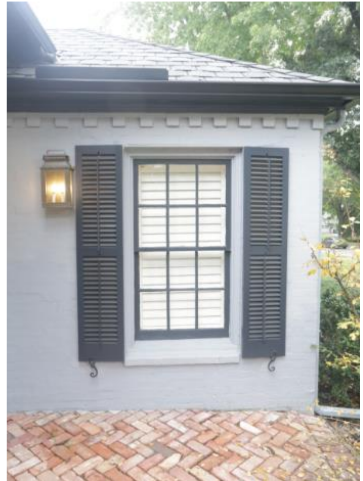
Above: six-over-six window, shutters, and brick detailing
