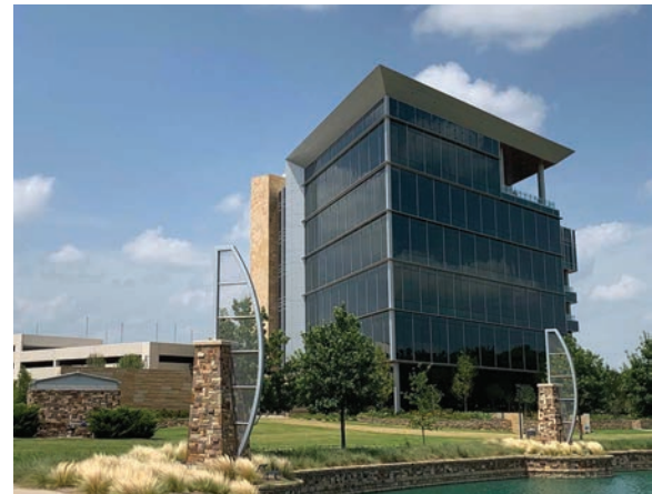
Office: Independent Financial (McKinney, TX)
