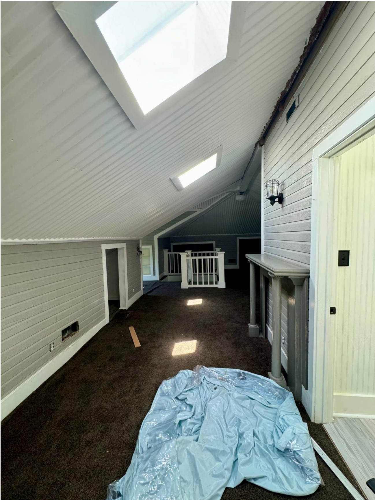
Secondary view of upstairs open area with period incorrect skylights. Tarp required to catch rain that comes through the roof.
