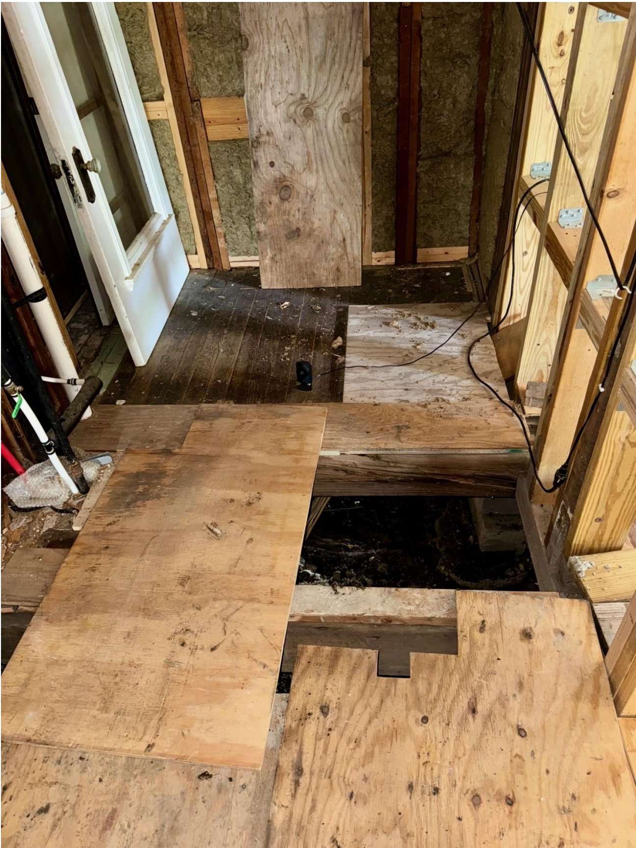
End of main hallway. Holes in the floor, most areas covered by plywood due to missing subfloor
