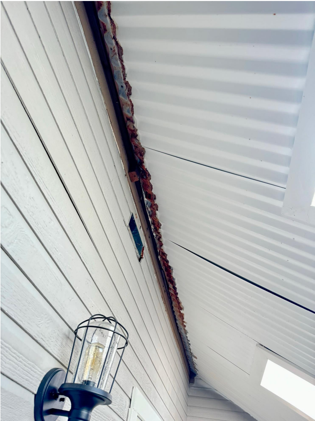
View of upstairs ceiling condition and continuing water damage due to failing roof
