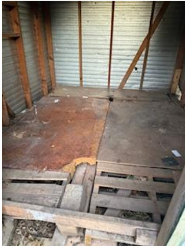
Above: Shed Interior showing rotted and missing floor
