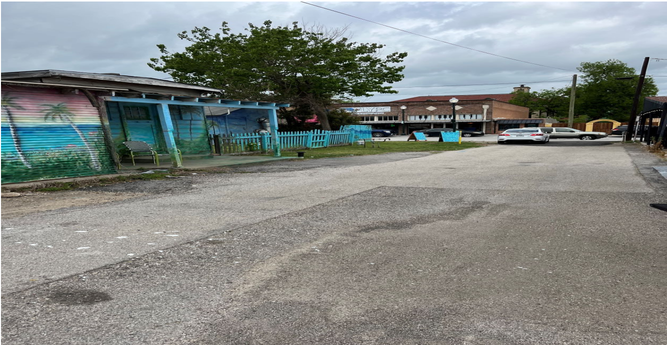
Alley – rear of 101 S. Chestnut facing Louisiana St.
