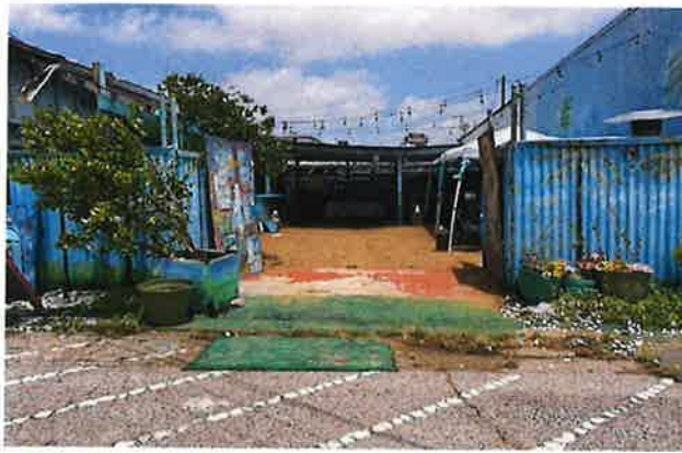
Existing front fence and gates
