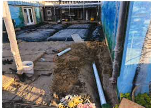
Relocate and extend wastewater drain from neighbor
