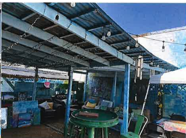
Existing patio cover slopes to center of patio space
