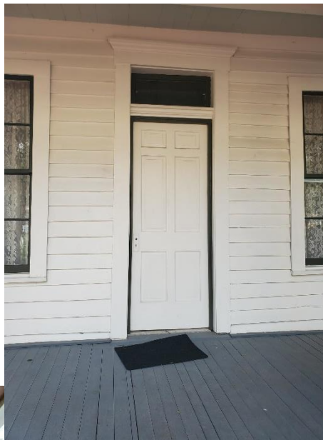
Door on the west side replacing the original chimney/fireplace
