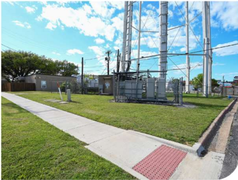
Existing View of Chestnut Tank
