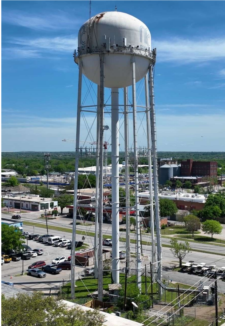
Existing View of Chestnut Tank
