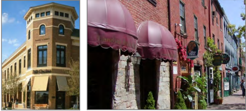
Buildings with architectural features and storefront elements that add interest along the street.
