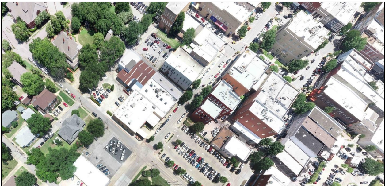
Figure 5: Drone Photo, Zones A and C
