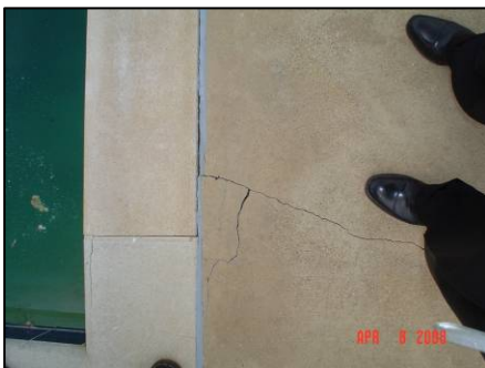
Movement Cracks in Deck
