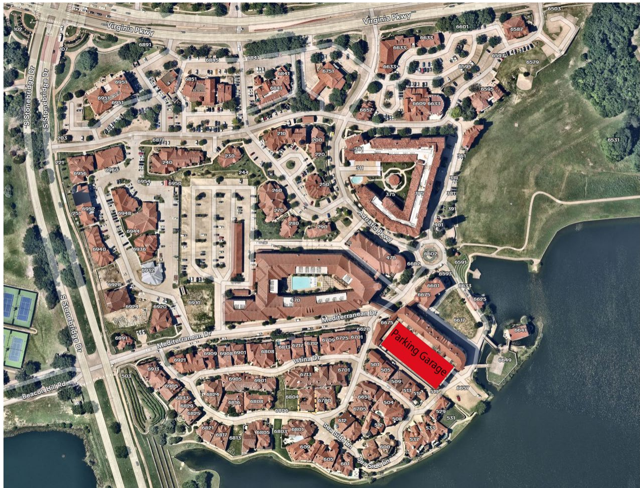
The Adriatica Village development is located on the Southeast corner of Stonebridge Drive and Virginia Parkway. The parking garage shown above provides parking for restaurants, retail shops, offices and visitors to the park and amphitheater.
