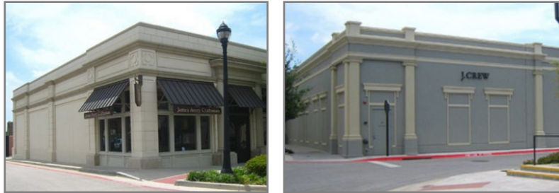
Images showing the side and rear facades buildings finished to match the color and materials of the front facades
