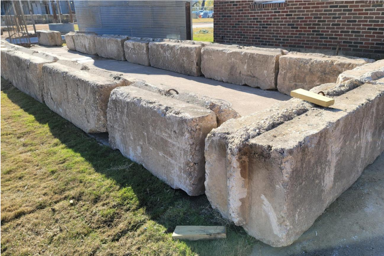
Concrete Blocks for Sign Base and Site Lighting for Sign Area
