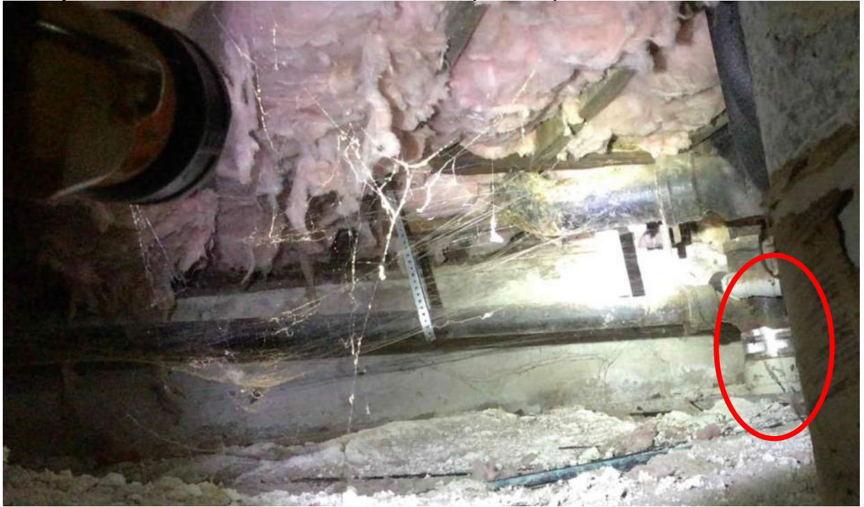
Examples of mixed PVC / cast iron sections (1-16-25)
