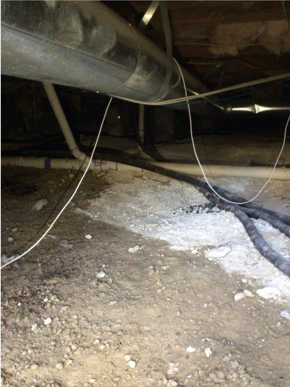
1-16-25 Evidence of leakage from current PVC sewer lines (1-16-25)
