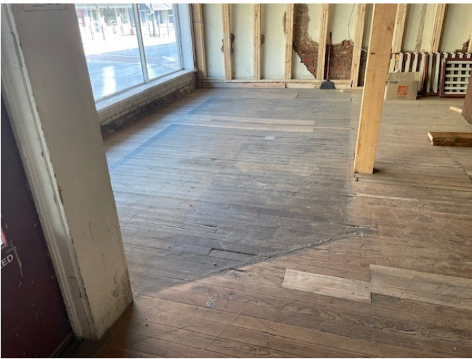
Repair of Damaged Floor
