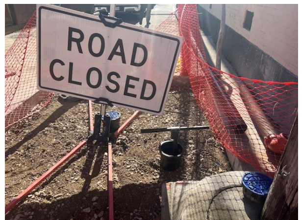
Installed water valve
