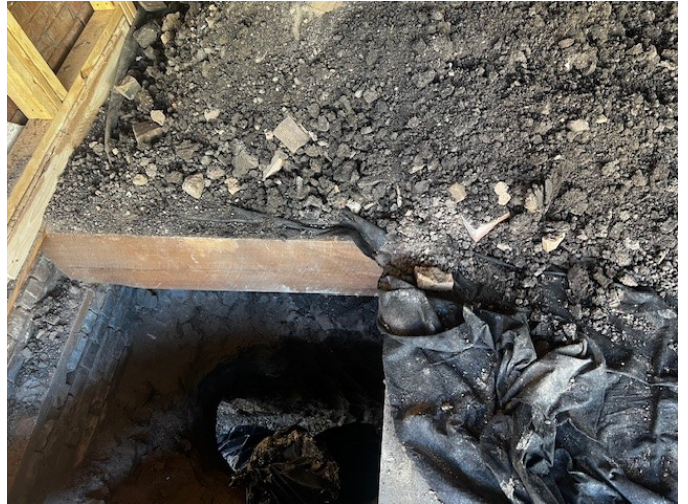
Create space to install water piper
