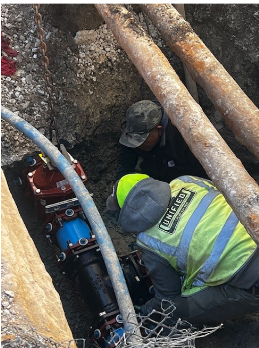
Install water main connection
