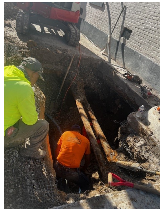
Locate Water Pipe
