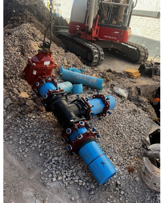
Install water main connection
