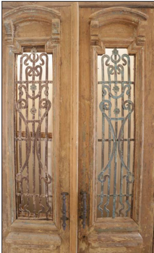
Wrought Iron Door Detail
