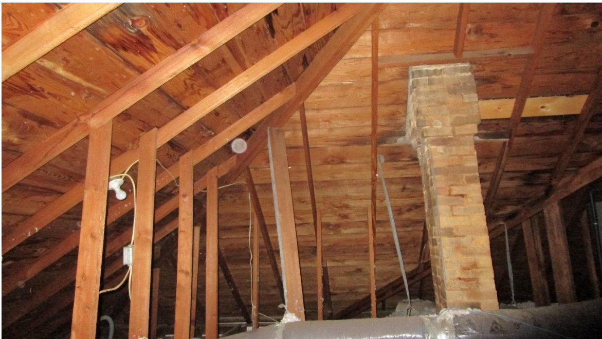
Photo #44 View of the attic framing looking to the northwest corner of the building.
