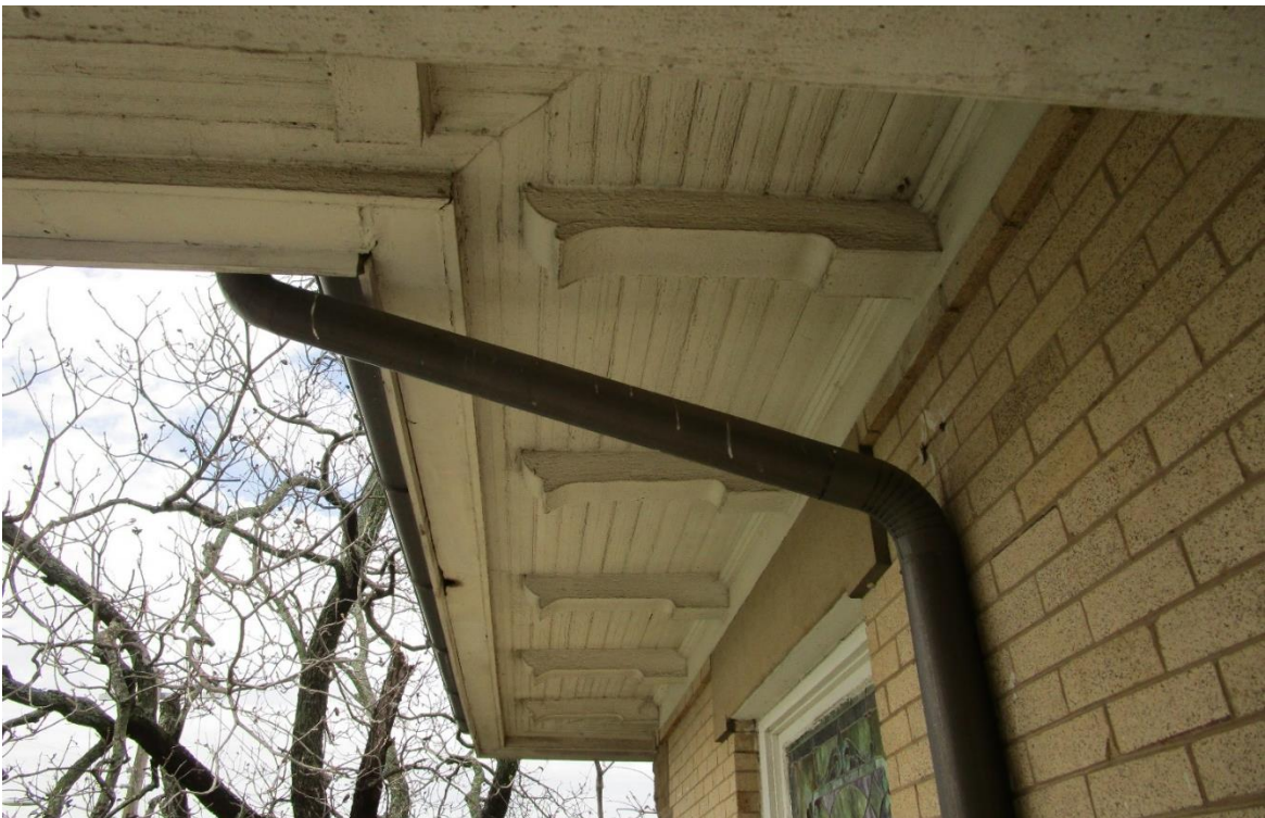
Photo #50 Underside of roof soffit on south side looking west.
