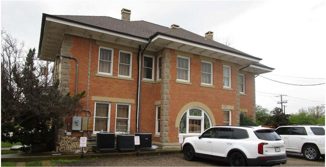
Photo #1 View of the north side of the building.
