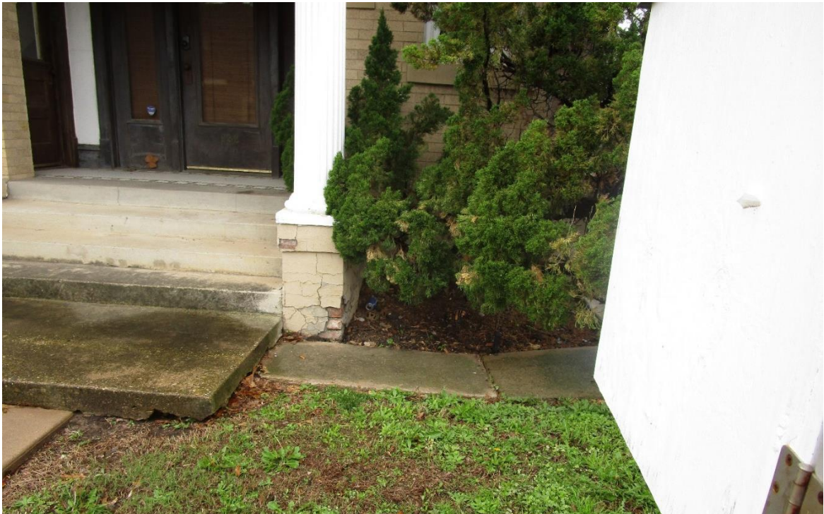
Photo #11 Stucco covered brick wall at north side of the east porch entrance.
