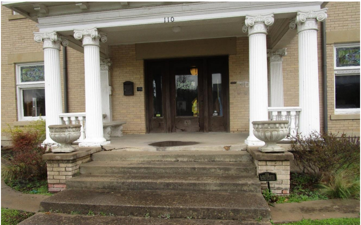
Photo #22 View of the lower level of the south entrance coverer patio.
