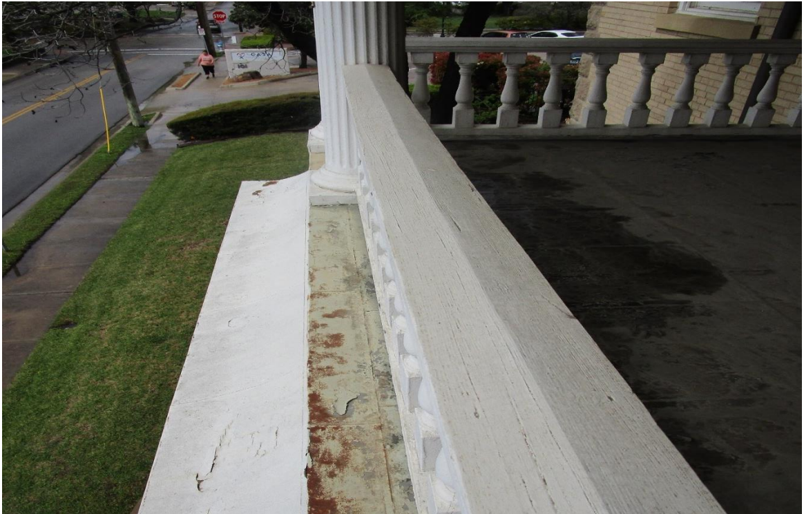
Photo #54 View of the south side of the lower roof for the entrance patio looking west.
