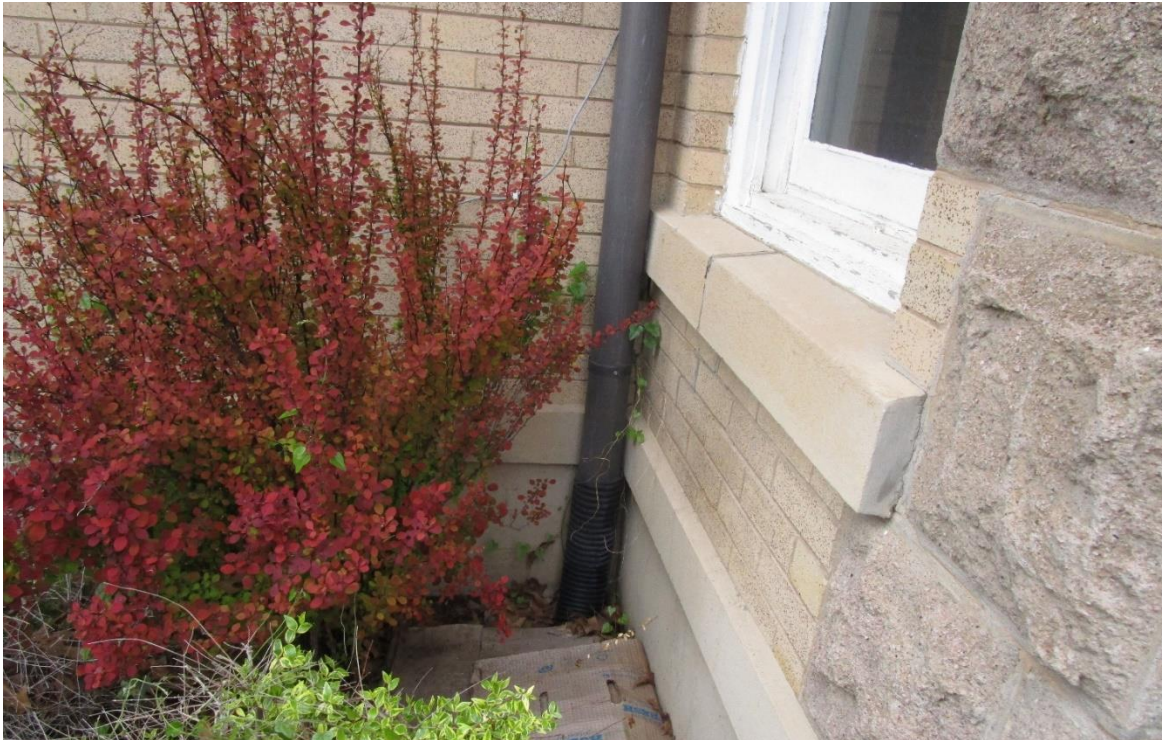
Photo #15 Downspout connects to underground pipe.
