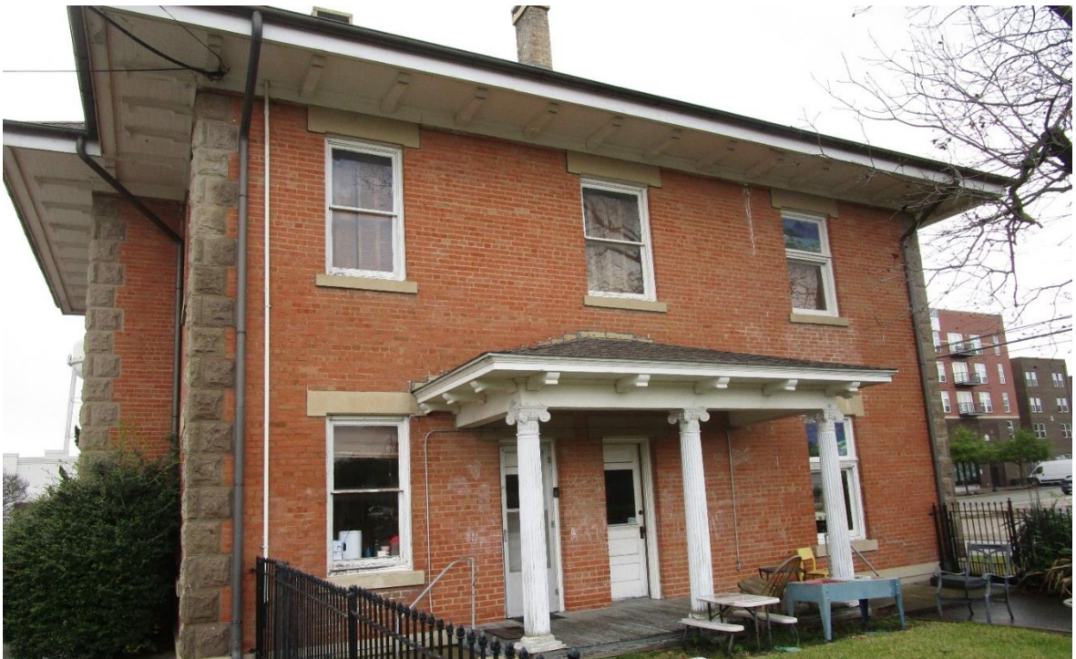
Photo #6 The west side of the building.
