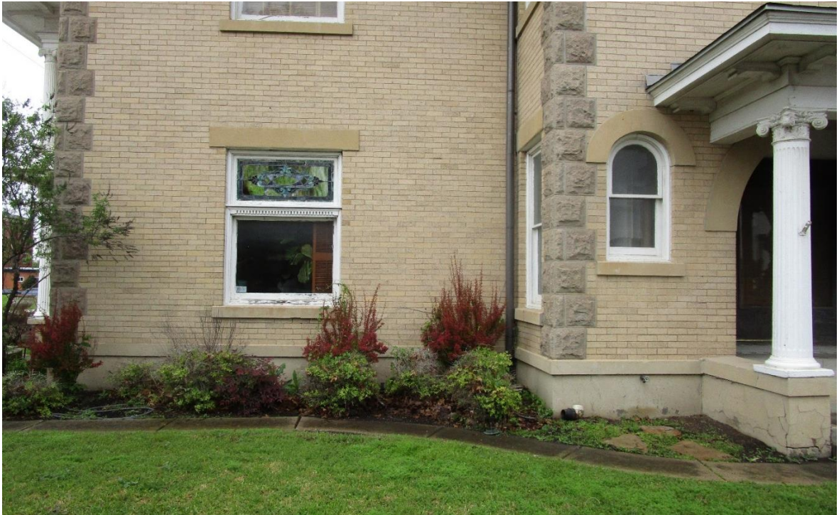
Photo #17 The east brick wall appears to be in good condition.
