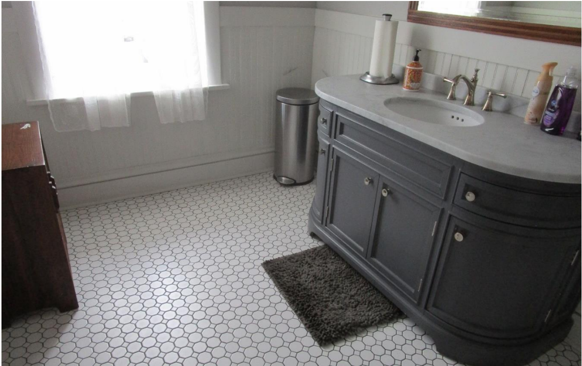
Photo #41 Upstairs bath room is in good condition.
