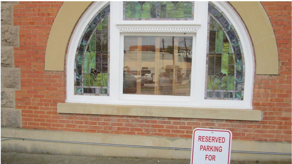
Photo #62 Window on the north side of the building.
