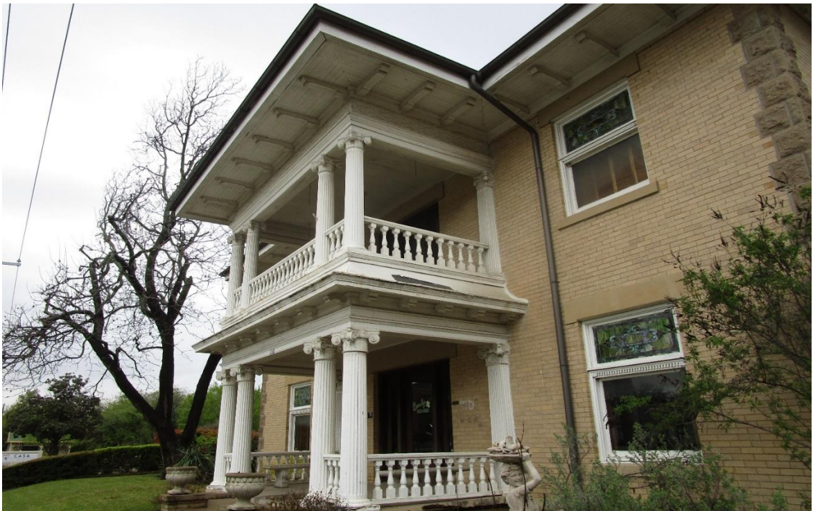
Photo #18 Two level covered porch on the south side of the building.
