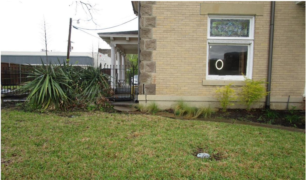
Photo #25 Southwest corner of the building.
