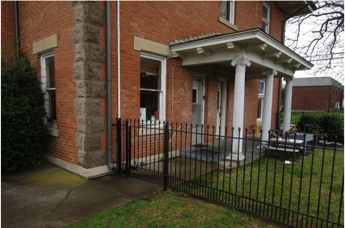
Photo #7 Northwest corner of the building.
