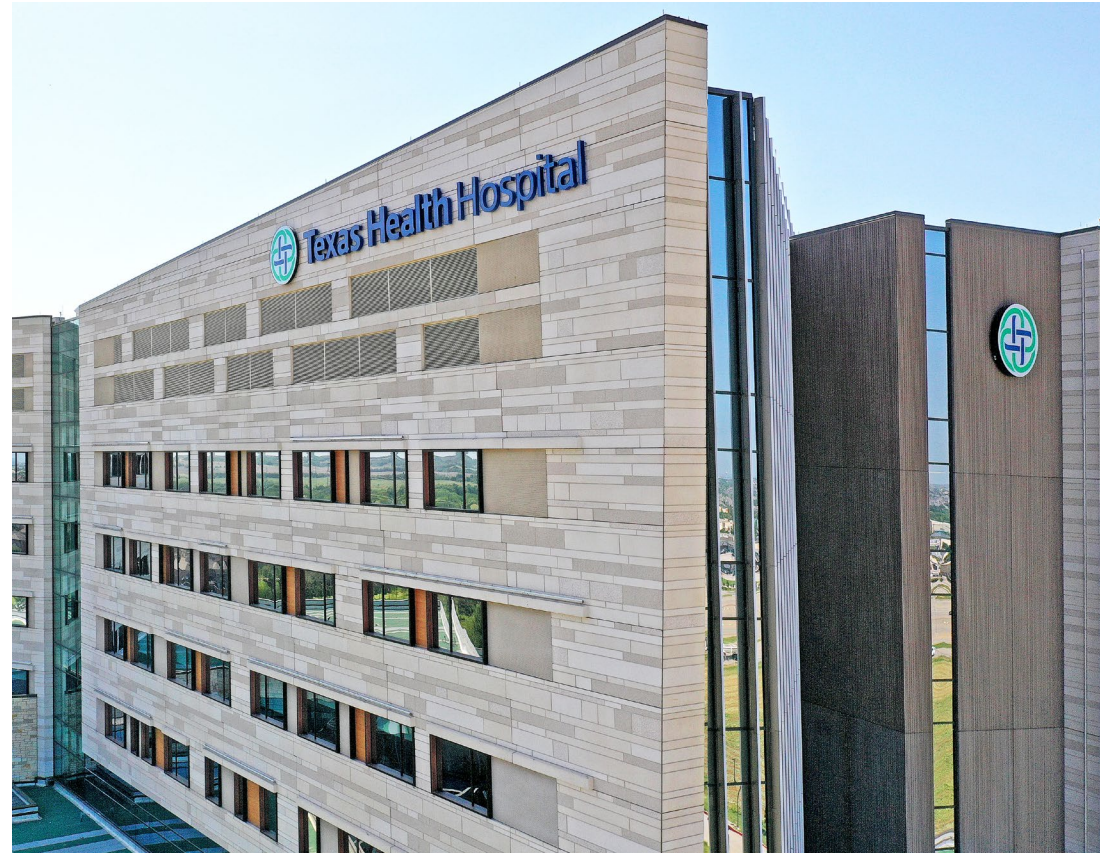
Texas Health Frisco Hospital – Custom Precast Panels to simulate look of natural stone
