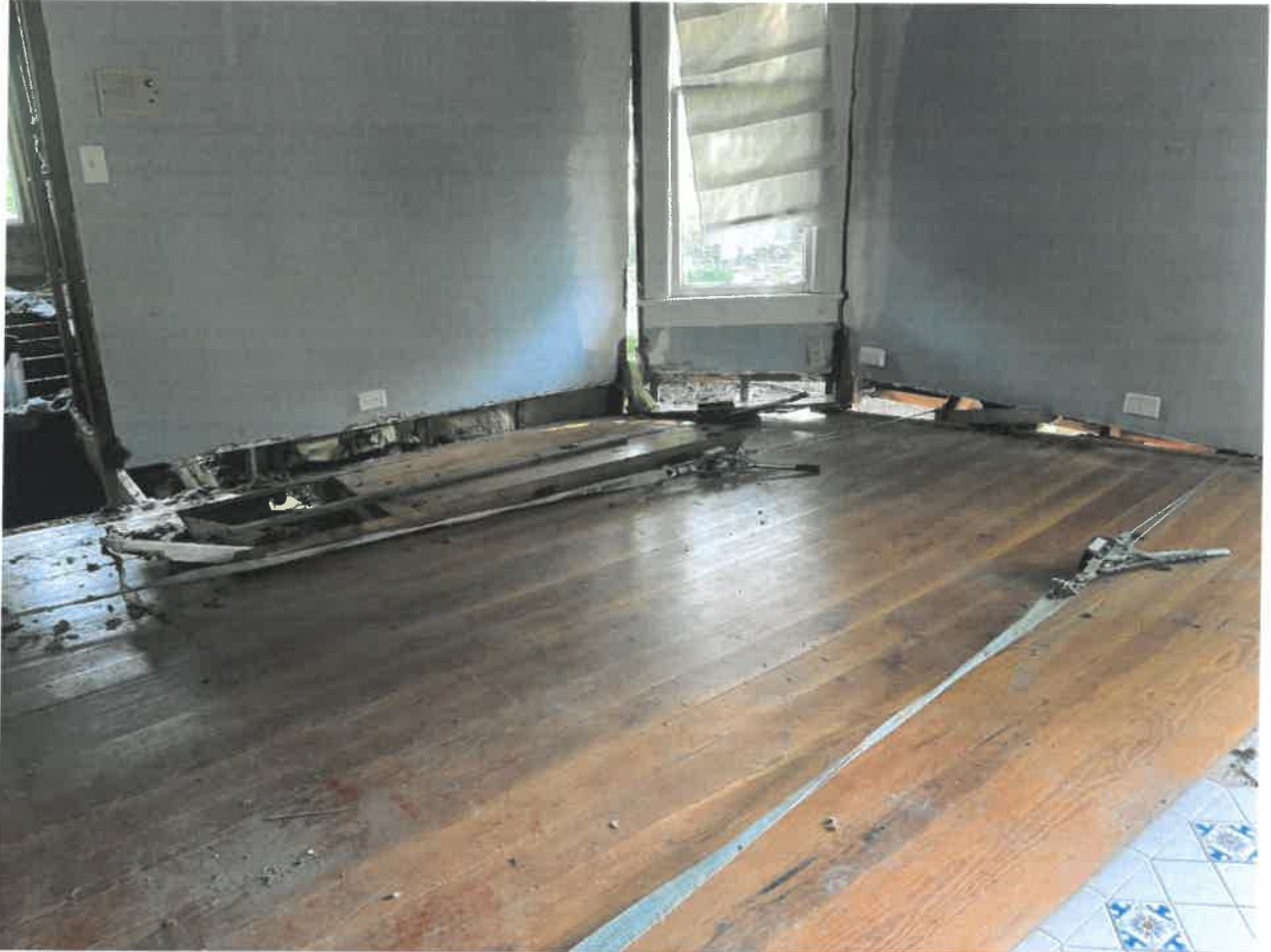
PHOTO 4 – INTERIOR FRONT LIVING ROOM SHOWING FLOOR SEPARATION FROM WALLS AND FRAMING DISTORTION
