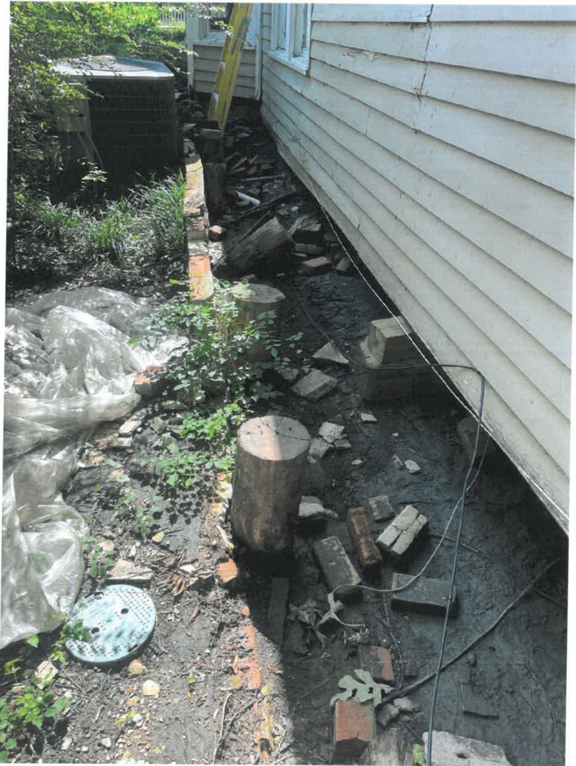
PHOTO 2 – NORTH SIDE OF HOUSE FOUNDATION WAS SUPPORTED ON BOIS D'ARC WOOD PIERS HOUSE SHIFTED TO RIGHT
