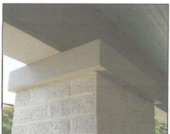
Plain limestone cap on brick column
