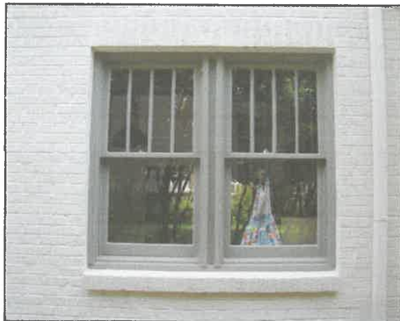
4-over-1 vertical proportioned windows
