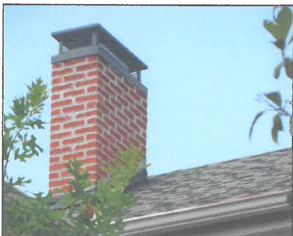
Chimney made of "carpet" brick
