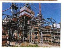
May 16 - May 20Remove tin off existing structure, demo canopies, drilling and pouring piers at Brewer
