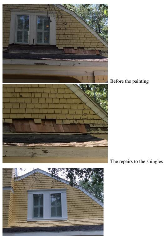
Photographs of Before/After Exterior Painting and Repair - Carriage House
