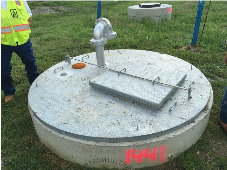
Typical Air Release Valve and Odor Control
