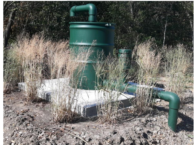
Typical Odor Control Canister
