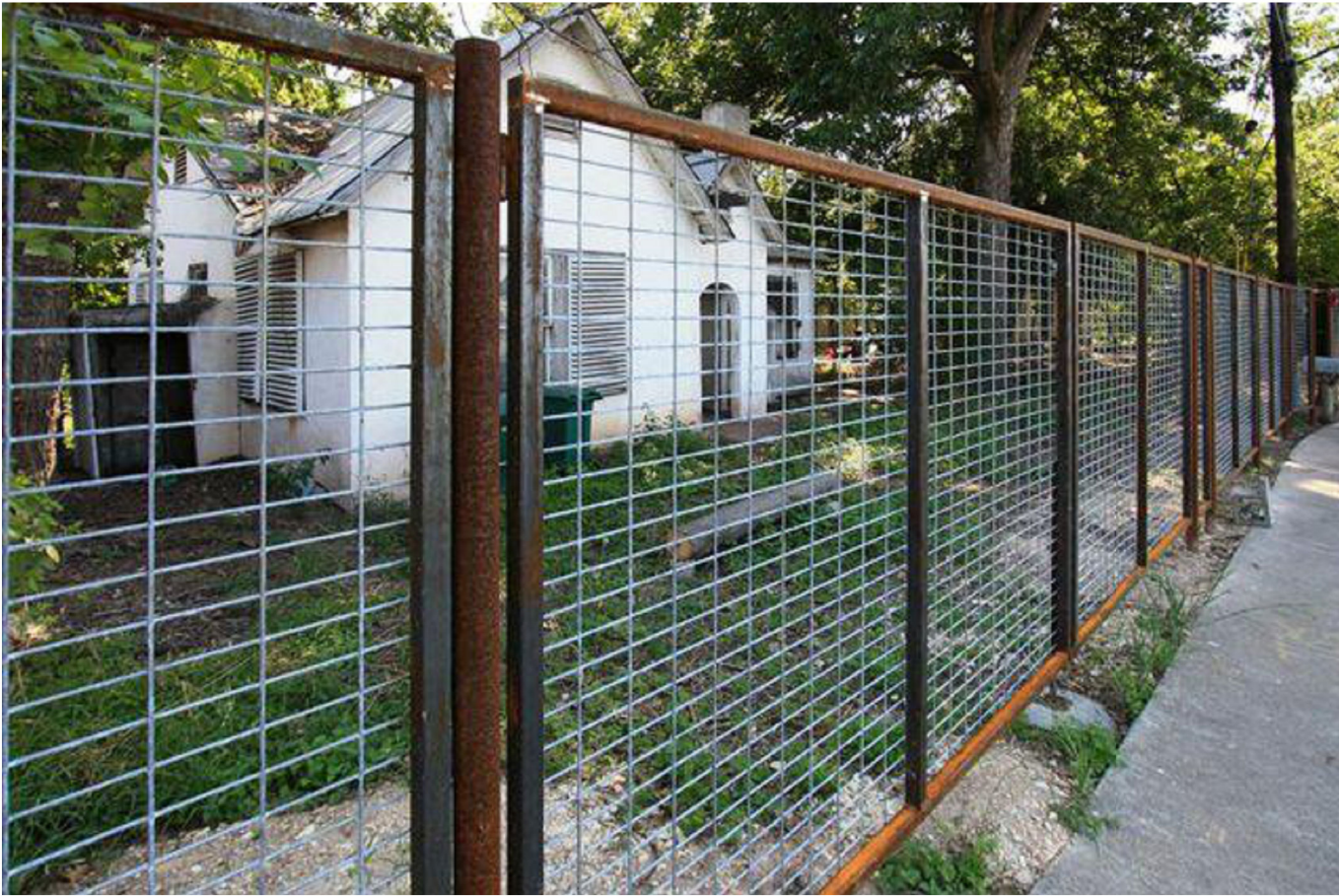
TYPICAL METAL FENCING AROUND SITE - STEEL POST WITH STEEL FRAMED WELDED WIRE FABRIC, HEIGHT VARIES 6' - 8' FENCING TO BE USED AS REQUIRED SCREENING ALONG REAR OF BREWERY (SOUTH END OF SITE) FOR HVAC EQUIPMENT AND OVERHEAD DOORS AND ALONG SOUTHEAST CORNER FOR OVERHEAD DOOR.
