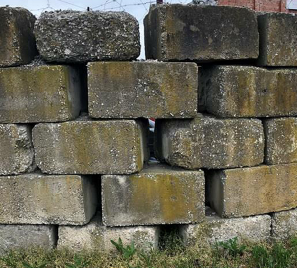
RECLAIMED CONCRETE BLOCKS FROM ADJACENT BIG BASS TOWING SITE 36" LONG X 18" HIGH X 24" DEEP BLOCKS STACKED 7'-6" HIGH USED ALONG EAST PROPERTY LINE FOR SCREENING AND SOUND MASS SOUND BARRIER TO RESIDENTIAL
