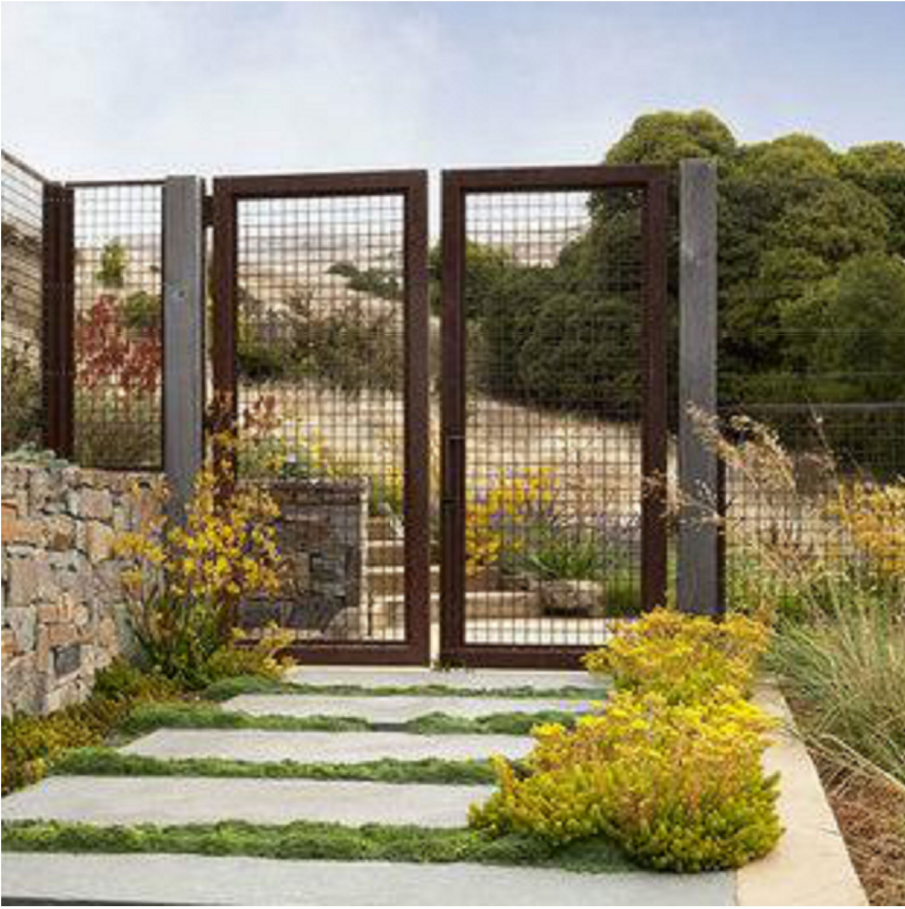
TYPICAL GATES IN METAL FENCING. STEEL FRAMED WELDED WIRE FABRIC, HEIGHT TO MATCH FENCE HEIGHT.
